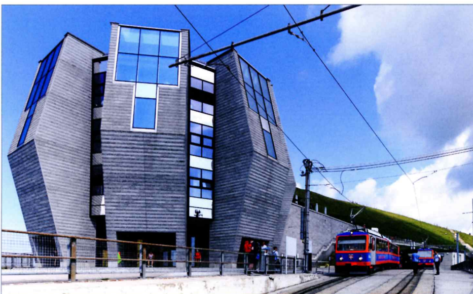
The Generoso Vetta terminus is dominated today by the "Fiore di pietra", the new summit restaurant. Photograph taken 21 August 2021.
