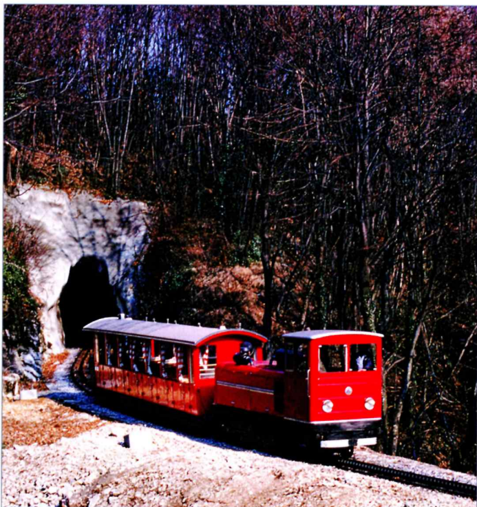
On 21 March 1981, Hm 2/3 No.1 propels a panorama car uphill. In view of the forthcoming electrification, the tunnel visible in the background has been widened and lined with shotcrete.
