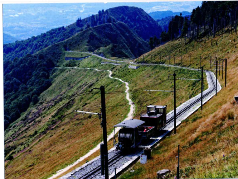
In dry weather, an auxiliary train for the fire brigade runs behind each steam train in order to extinguish any fires on the embankment as quickly as possible. Auxiliary train with the Hm 2/3 No.1, was photographed below the Generoso Vetta mountain station on 21 August 2021.
